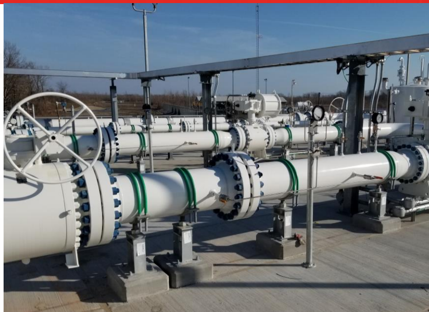
Trunnion-Mounted Ball Valve
