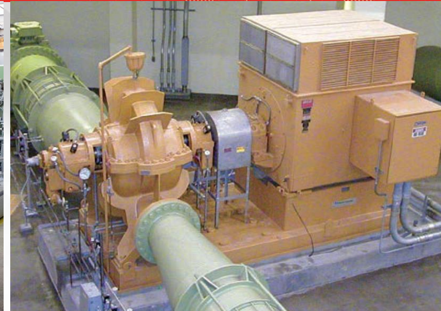
Single-Stage Pipeline Pump
